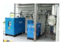
Biogas screw compressor and treatment system equipment for Biogas Power Generation in Beijing Landfill Site
